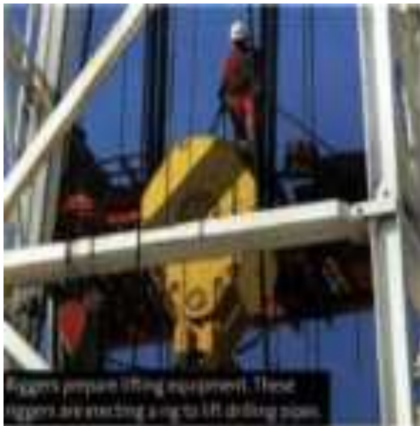
Riggers also work with crane operators. First, they attach slings to a load. Then the crane lifts the load.
